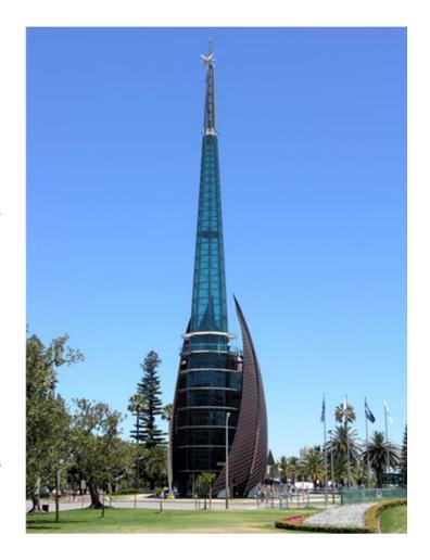
made with reinforced concrete cast in situ. Soundproof louvres and doors are used to muffle or direct the sound towards the city, or the river, as required. The glass-clad spire is designed using spokes which radiate horizontally from a centrally positioned axle, declining in width as it rises to a point. The solid-steel columns of the spire are rectangular, and the concrete bell chamber is enveloped in 30 metre high (98 ft) copper sails and glass.
